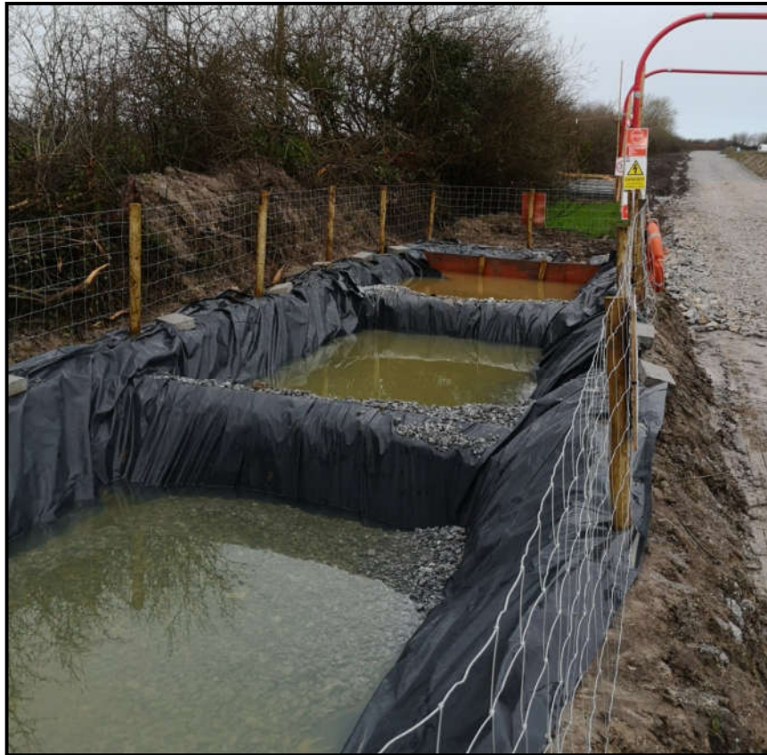
Figure 3—3 Multi tiered settlement pond with stone filter installed during construction works
