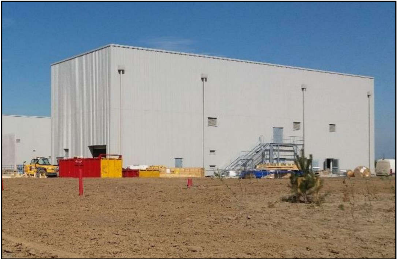
Figure 3—5 Typical finished GIS substation building
