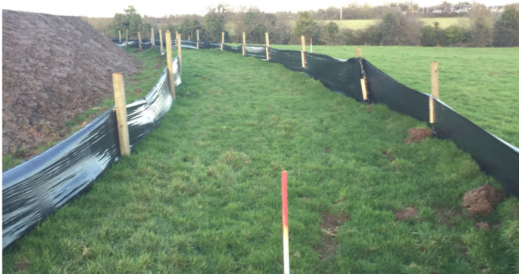
Figure 3—4 Hy-Tex Terrastop silt curtain fencing installed around temporary deposition areas
