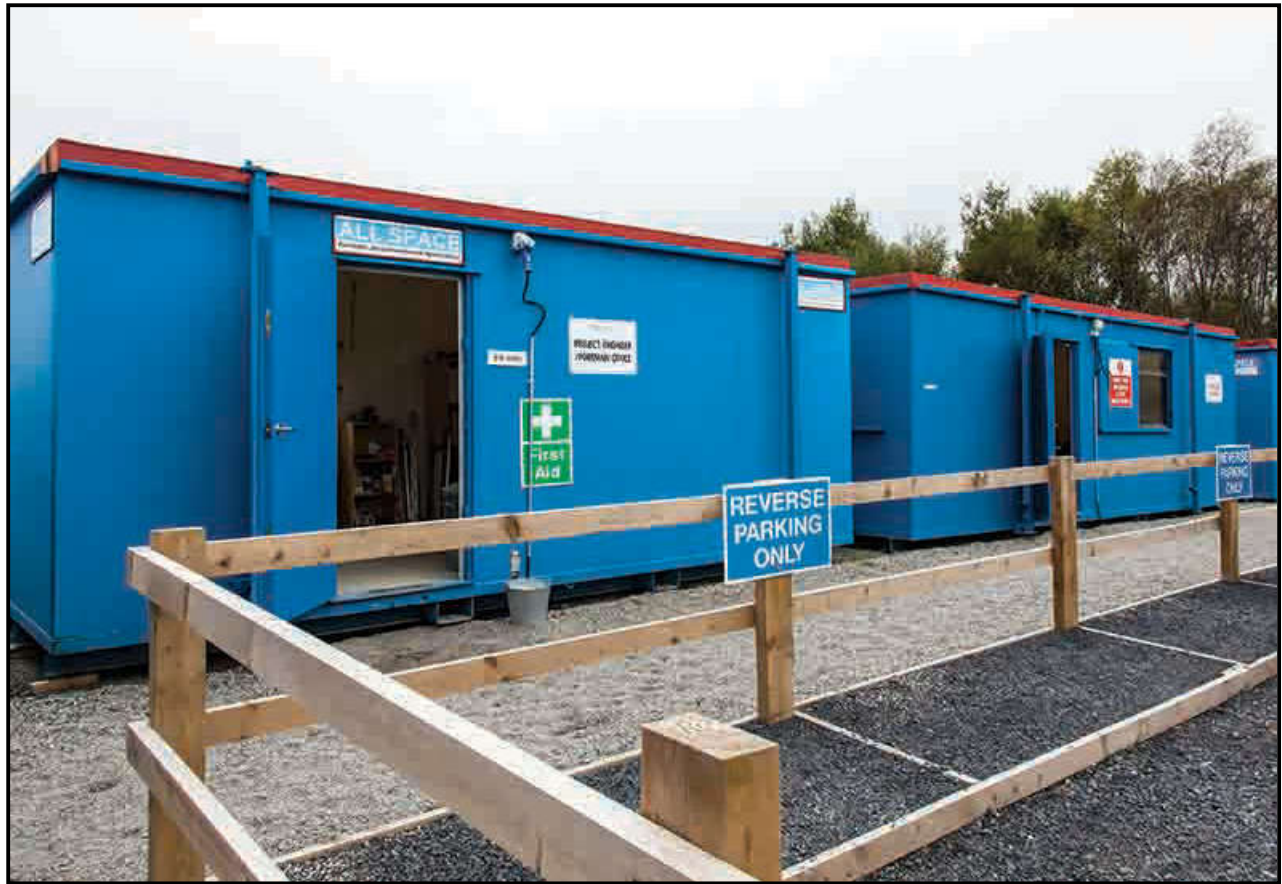
Figure 3—1 Typical temporary site construction compound
